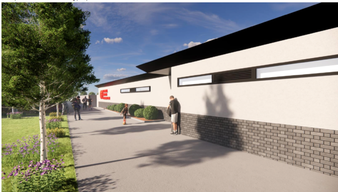
Visualisation 2: Proposed Clubhouse. Front. Contemporary design with render and brickwork facing on external walls. Flat roof with the potential for sustainable technologies such as PV panels and rainwater harvesting (TBC).
